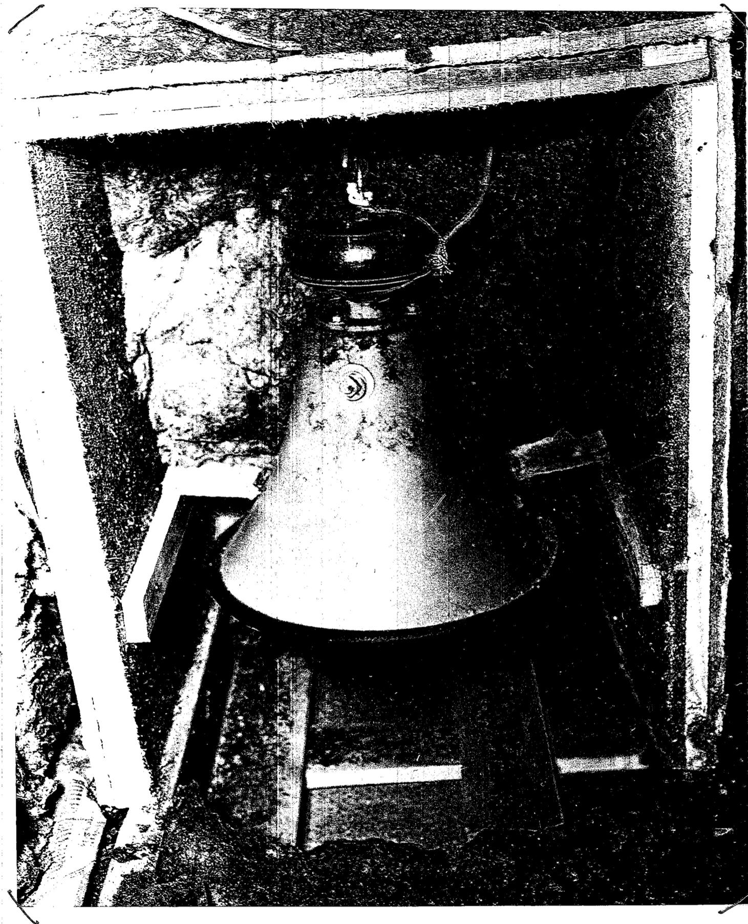
Microphone installation showing sound-proofing and position relative to ceiling. Celotex immediately below horn is the ceiling of the POW room below.
