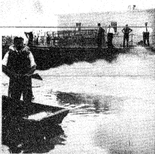
Navy's new method of eliminating fire hazards employs blowing treated sand over surface of oil slick.
